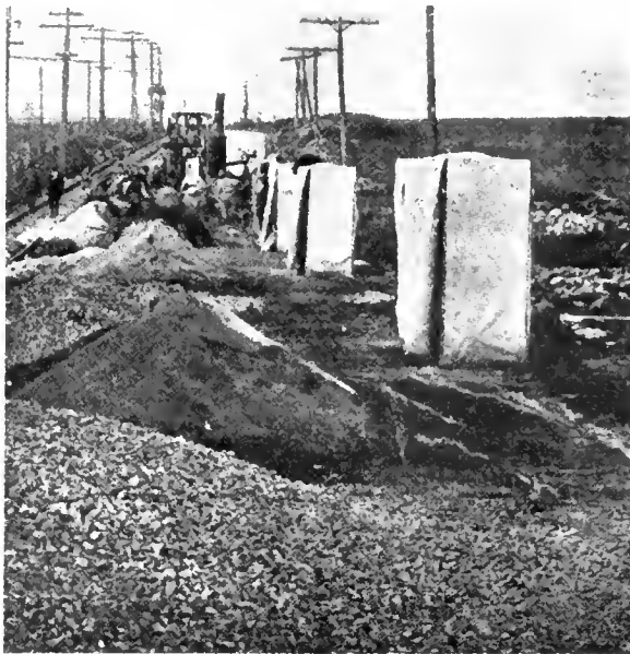
Philadelphia Model Highway Construction—Canvas Huts for Sheltering Cement.
